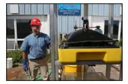
"1st phase fill": Operate fill pump until pressure gauge located on pump discharge achieves discharge pressure of Geotube circumference 30' circ 2.6 psi \* 45' circ 3.0 psi \* 80' circ 3.5 psi
